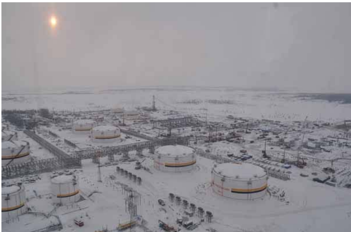
Oil treatment and water discharge facility "South"
